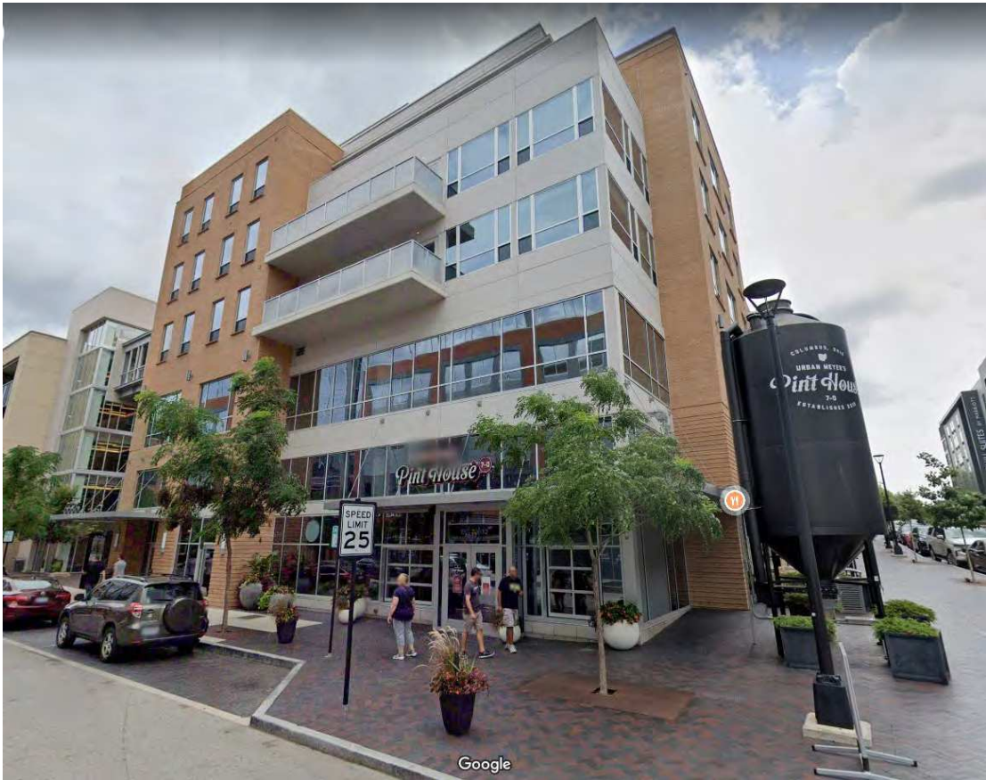
Figure 2: 6636 Longshore Street West Corner
