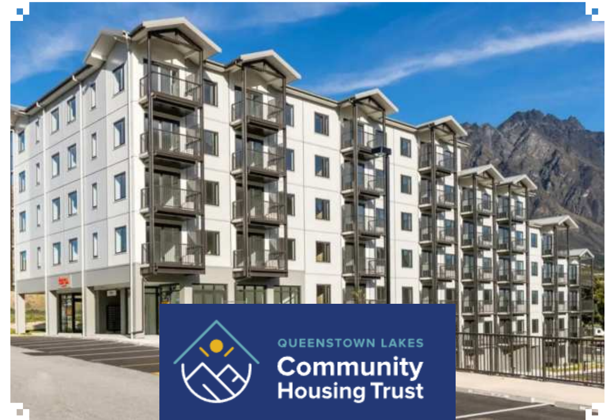
Figures 29: Toru Queenstown Community Housing Trust Note: (Queenstown Lakes Community Housing Trust, n.d.)
