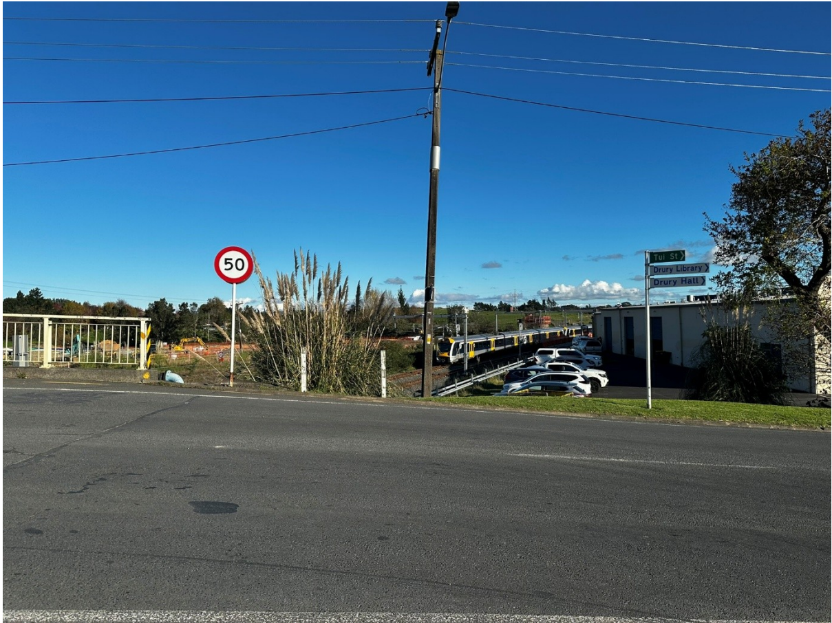
Figure 3: Train on the Southern Line, near Drury
