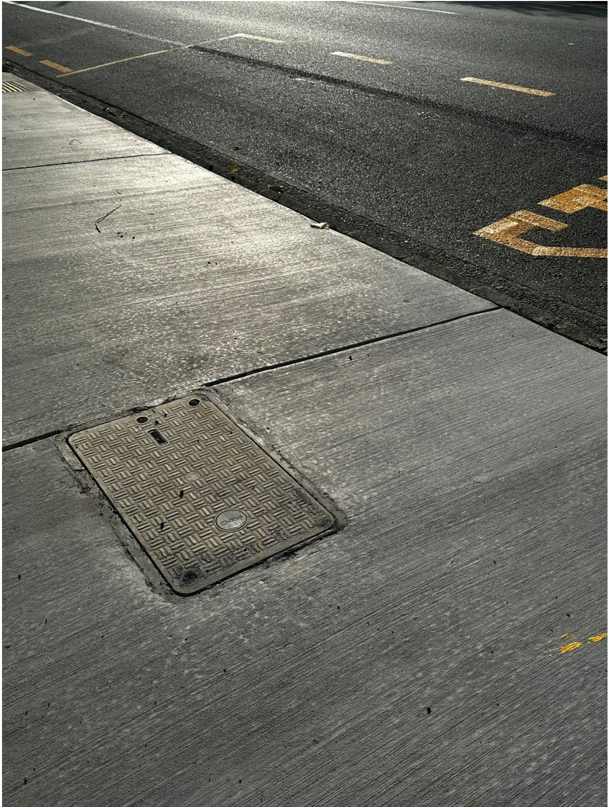
Figure 1: Chorus maintenance cover
